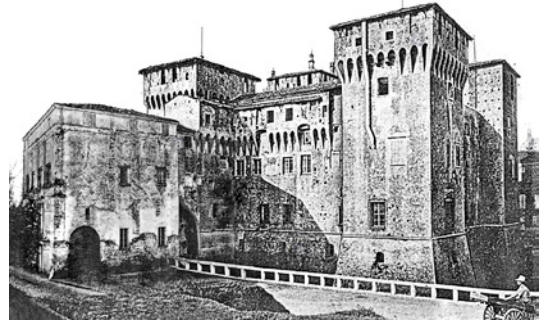
2. Mantua, Palazzina della Paleologa, now demolished. Photo author's archive.
