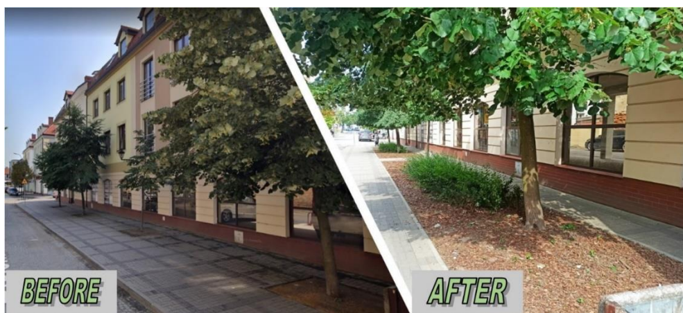
Fig. 2. De-concreting on Bielska Street in Płock
