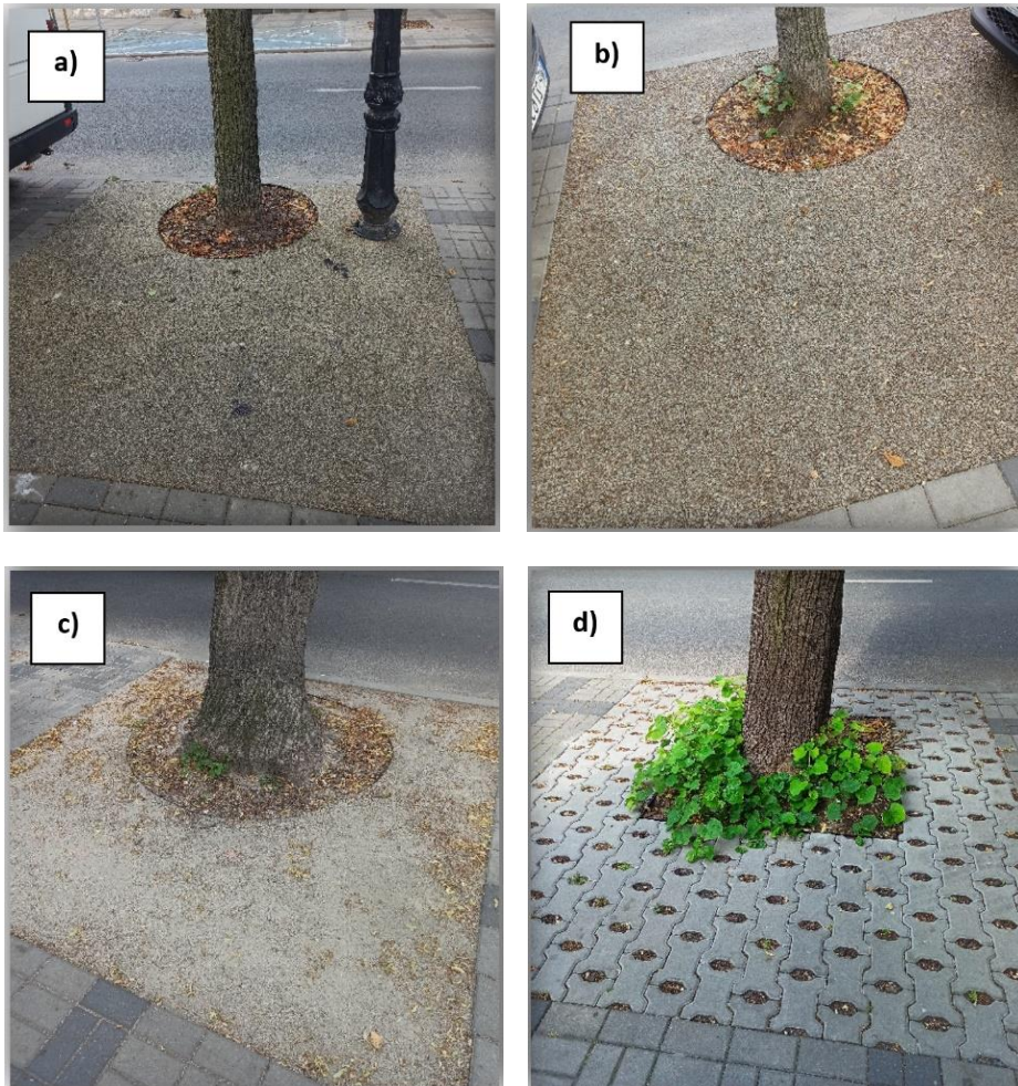
Fig. 3. Example of the application of surfaces a) TerraWay, b) EKOWAY, c) HanzaVia, d) Domino Eco on Kazimierza Wielkiego Street in Płock
